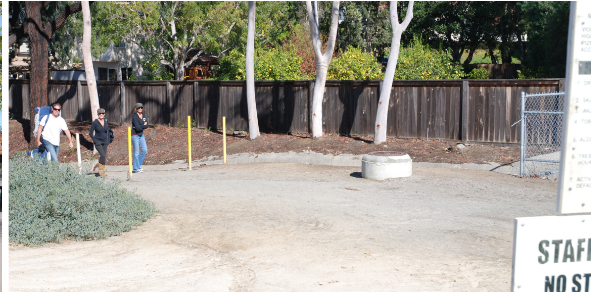
View of pathway to school's athletic fields. This more closely shows the lack of a defined inviting entry and is not ADA compliant due to the lack of paving and proper slope.
