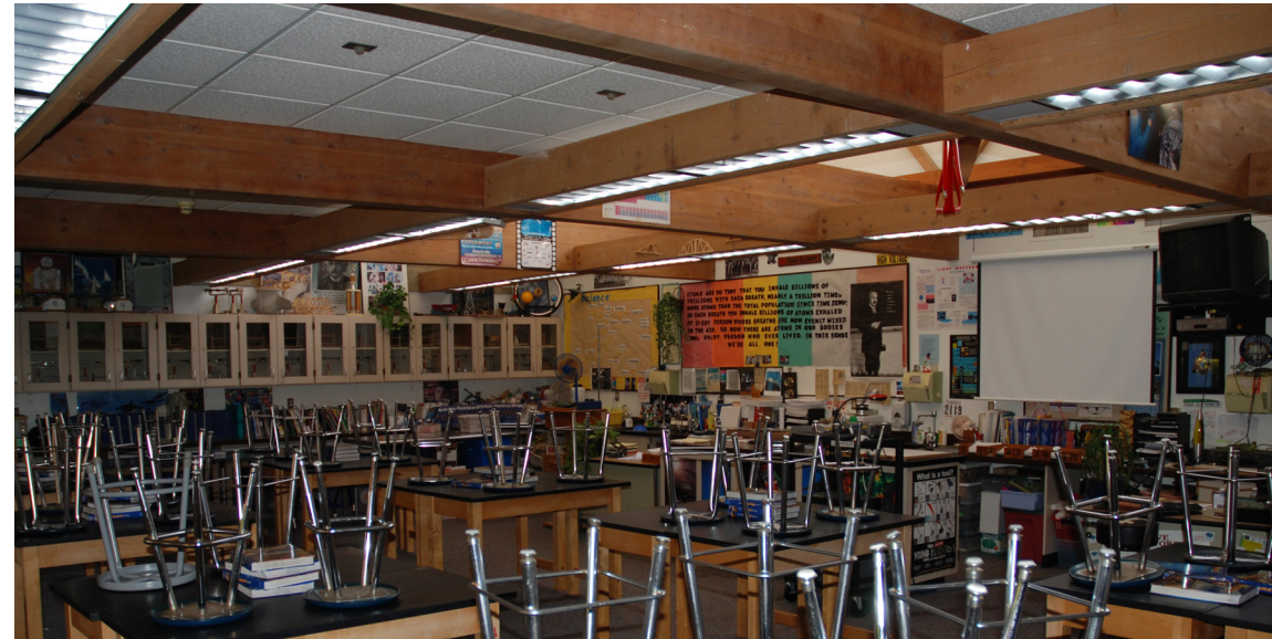
Interior view of typical science classroom. This shows the low ceiling height in the classrooms, which makes it difficult to add new power, data, lighting and upgrade HVAC in the exposed ceiling areas.
