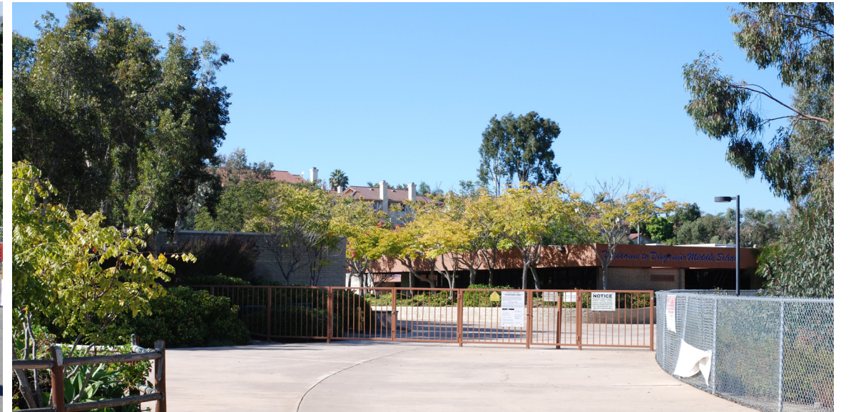
View of main gate entry into the campus.
