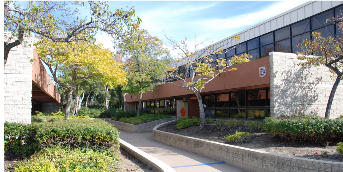
View of courtyard between typical classroom buildings.
