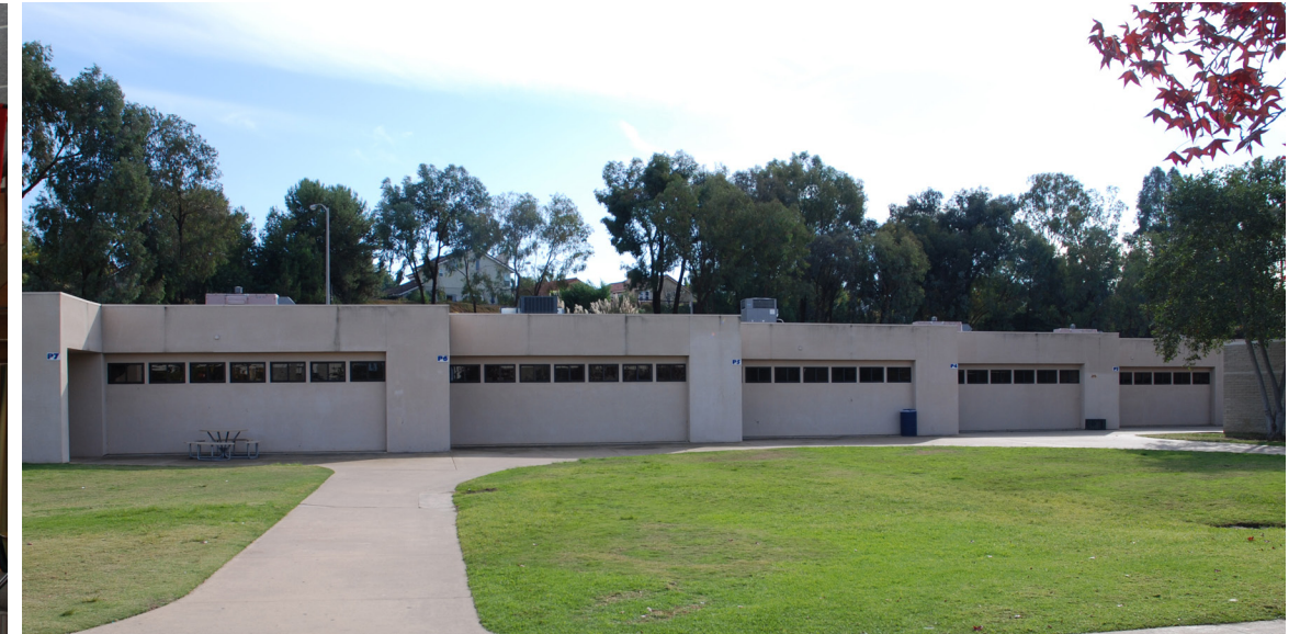
View portable classroom building on south end of campus. These classrooms have reached it useful life and needs to be replaced.
