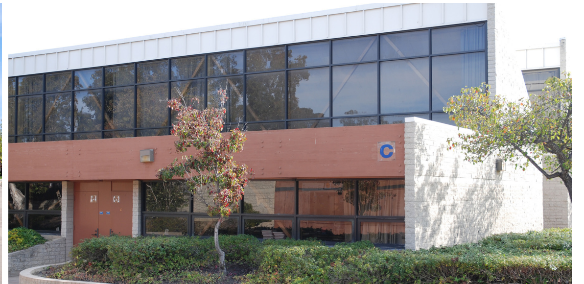
Closeup view of clerestory windows and entry. This high clerestory glazing makes it difficult to black out the rooms for video presentations.
