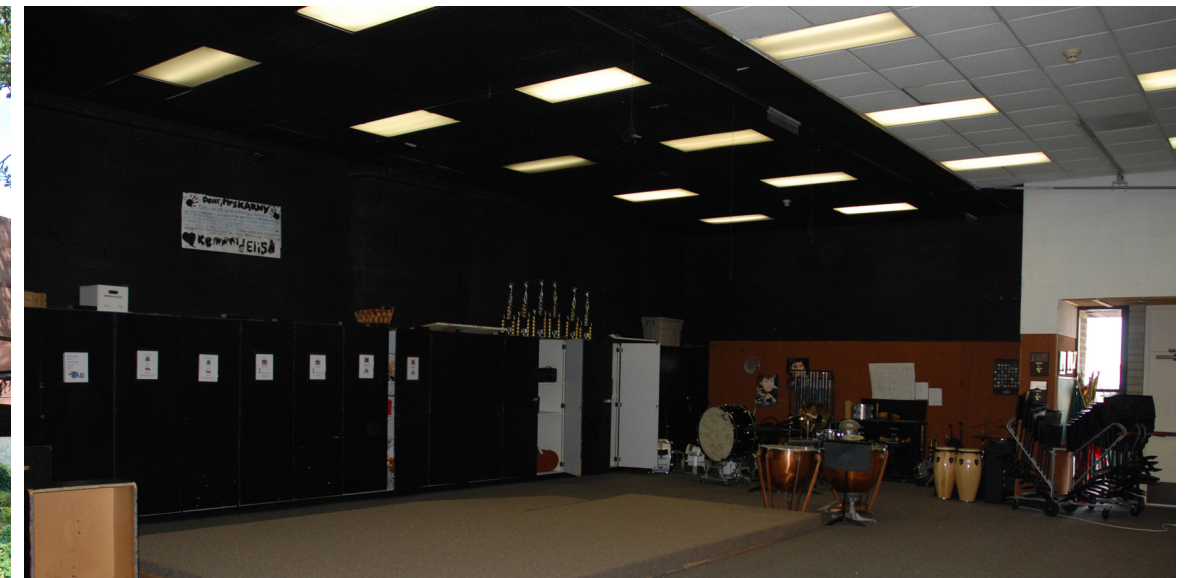
View of Cougar Hall area being used for band room and instrument storage. Very little acoustical quality in room. It is separated from the main multi-purpose area by an folding partition, which is not an acoustical solution.
