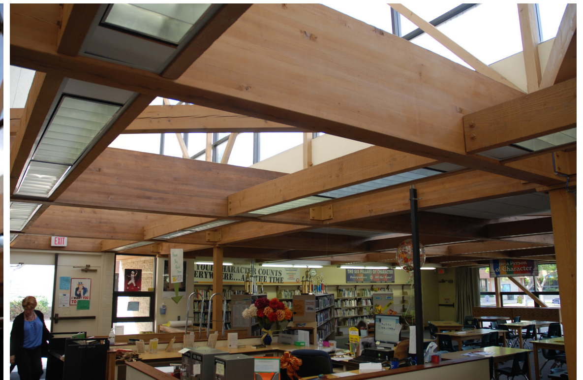
Closeup view of clerestory windows and beams in Media Center.
