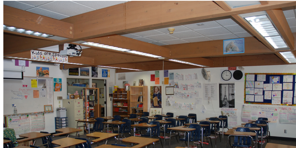
View of a typical classroom. The classrooms all have typical low ceilings.
