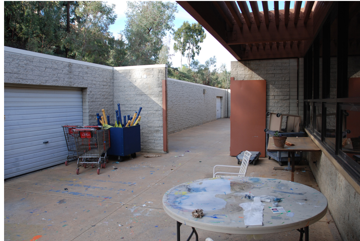
View of outdoor courtyard part of art classrooms. A very useable space when this building is converted for ASB, Art and C Smart.
