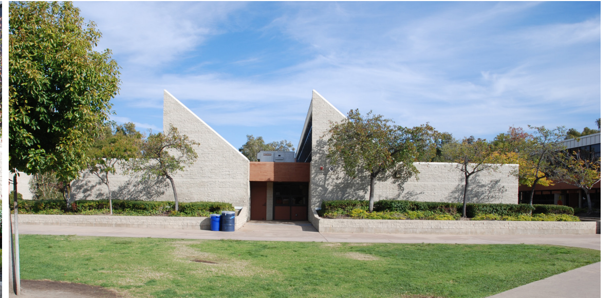
View typical classroom building showing the clerestory window forms.
