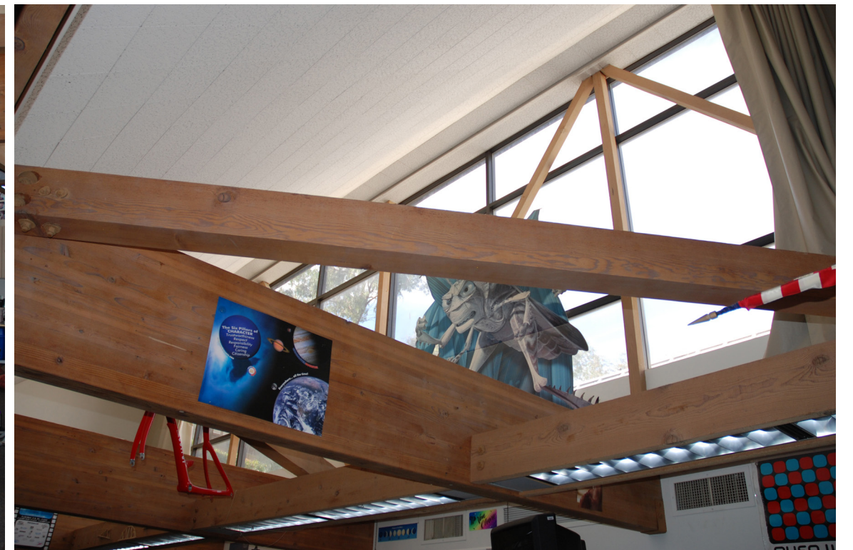
Detailed view of clerestory window in science classroom.
